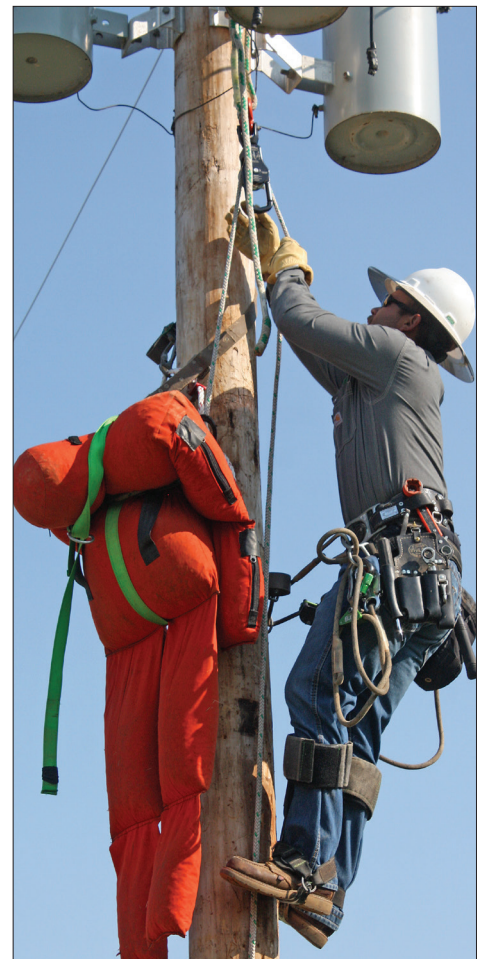
Top: ECE Lineman Lael LaBlanc secures the mannequin with a rope/pulley system during ECE's annual pole top rescue training. Once secure, he will cut the safety belt and lower the mannequin to the ground. PHOTO/AMY NIX, ECE.
