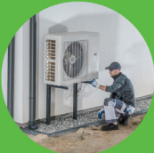
Air Source and Mini-Split Heat Pumps
